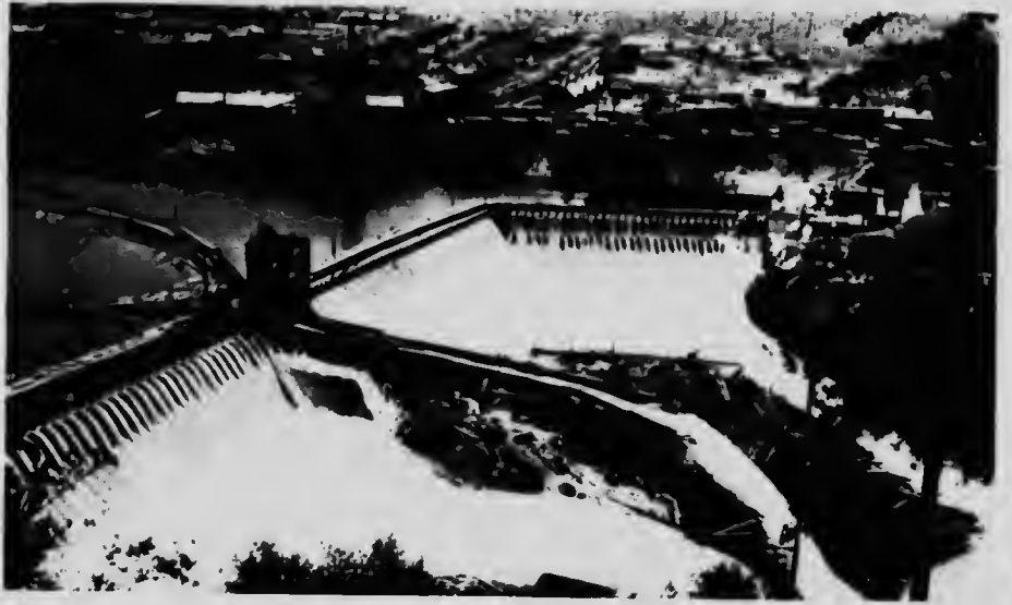
Powell River Development. Dam and Intake Works. Powell River.
